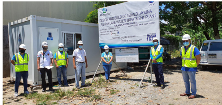
Poblacion WTP, also known as Laguna Lake Water Treatment Plant, during site inspection with MWSS
