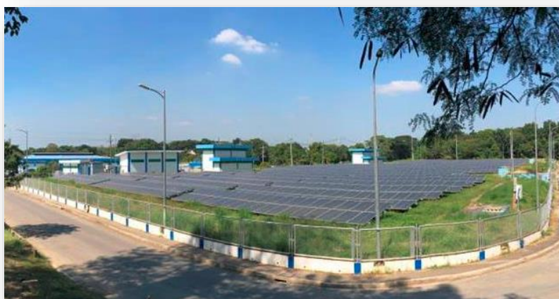
Photo of Maynilad Solar Power Plant (front view)
