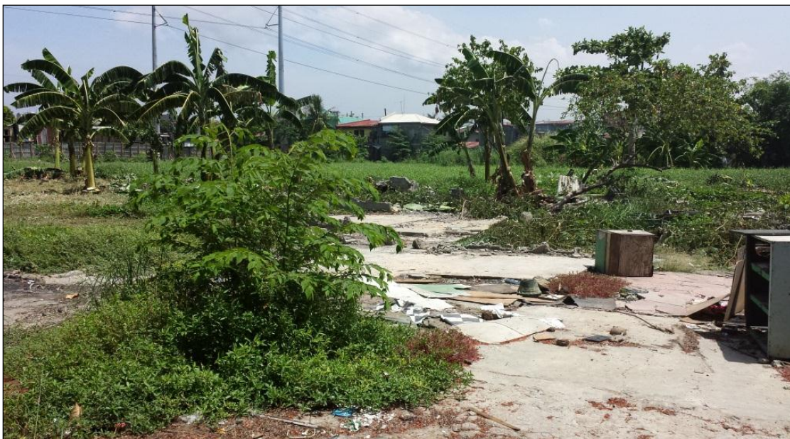
Figure 17. Photos of the clearing and fencing of the 3 properties acquired
