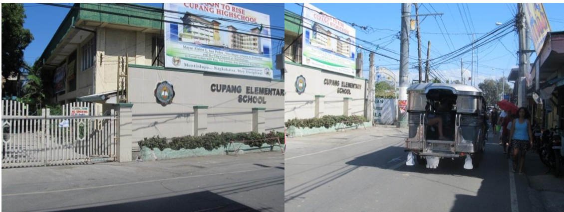
Figure 12. Frontage of Cupang Elementary School located along Manuel L. Quezon Street
