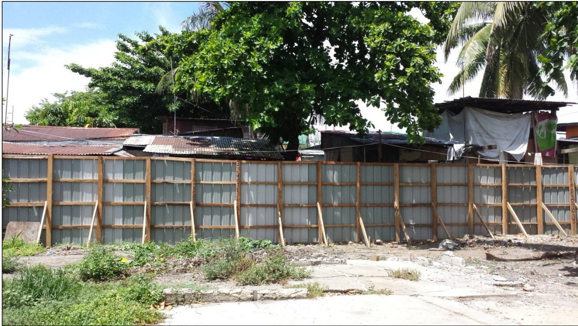
Figure 20. Property fenced to protect informal settlers located outside of the fence
