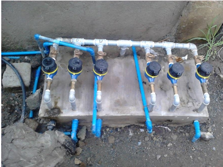
Figure 34. Six (6) new watermeters installed on-site as replacement for the DPs disconnected utilities.
