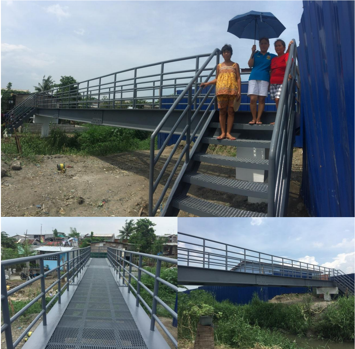
Figure 35. The newly constructed footbridge for access of the relocated households
