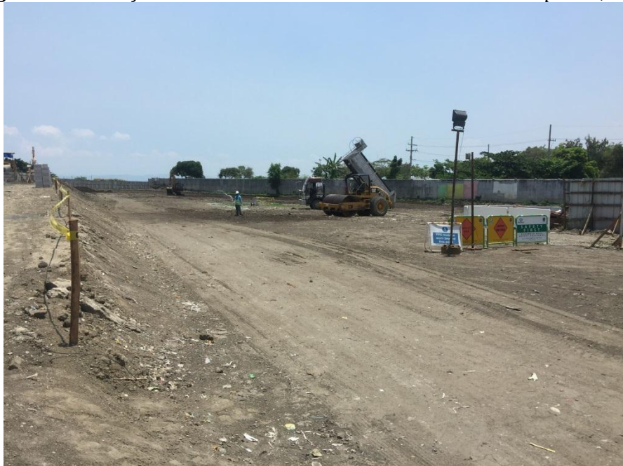
Figure 23. View of the site with installed fences
