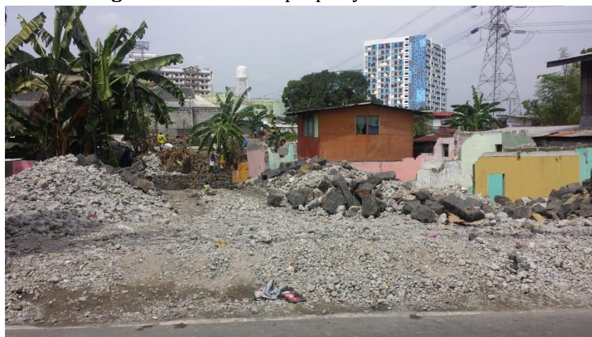
Figure 4. View of the property after demolition
