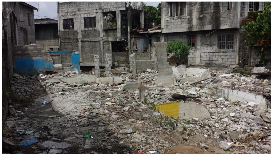
Figure 11. View of the property after demolition
