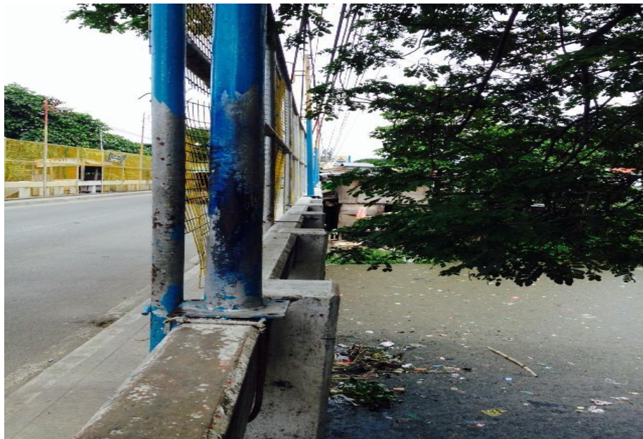
Figure 18. View of the side of Pasong Diablo bridge where the bridge crossing pipe will be installed
